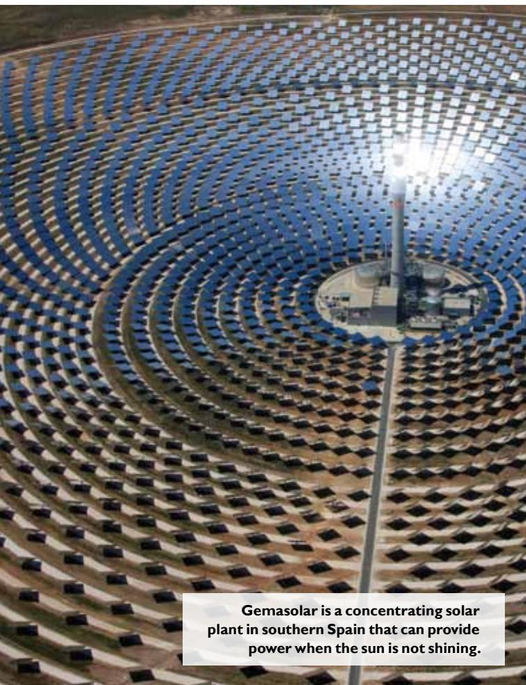
**Gemasolar is a concentrating solar plant in southern Spain that can provide power when the sun is not shining.**
